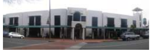
Figure 05: Steps in the façade and the roofline create projecting bays that break down the scale of a long building face
