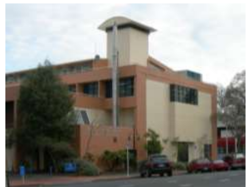
Figure 23: This side wall has some openings but for a public building presents a largely blank face to the street.
