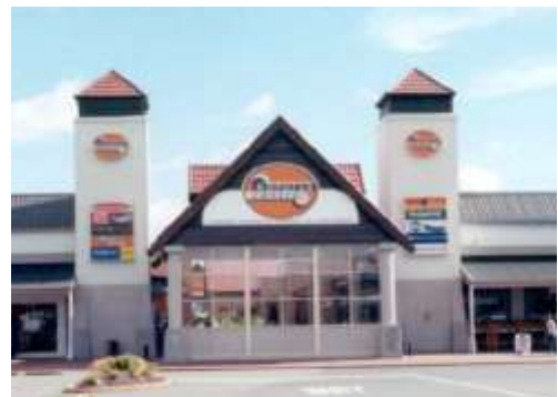
Figure 32: The turrets at Rotorua Central are not bad in their own right but overuse throughout the City Centre will devalue the form.
