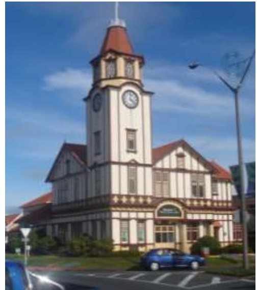
Figure 18: The tower at the Information Centre creates a landmark at the intersection of Fenton and Arawa Streets
