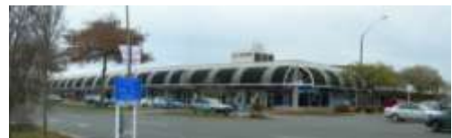
Figure 29: This building is reasonably large but the pilasters change the overall horizontal proportion to a vertical proportion to match neighbouring buildings. Note how the parapet line meets the cornice line of the building to the right, and the change of materials and capping creates a good top to the simple parapet structure.
